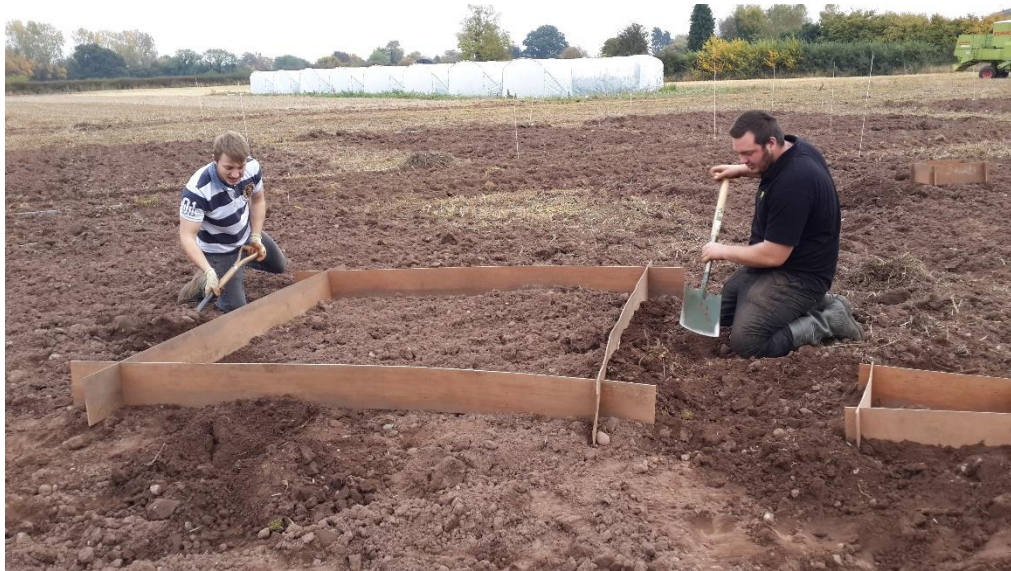
Figure 6. 11 Installation of the frame into the cultivated plots
