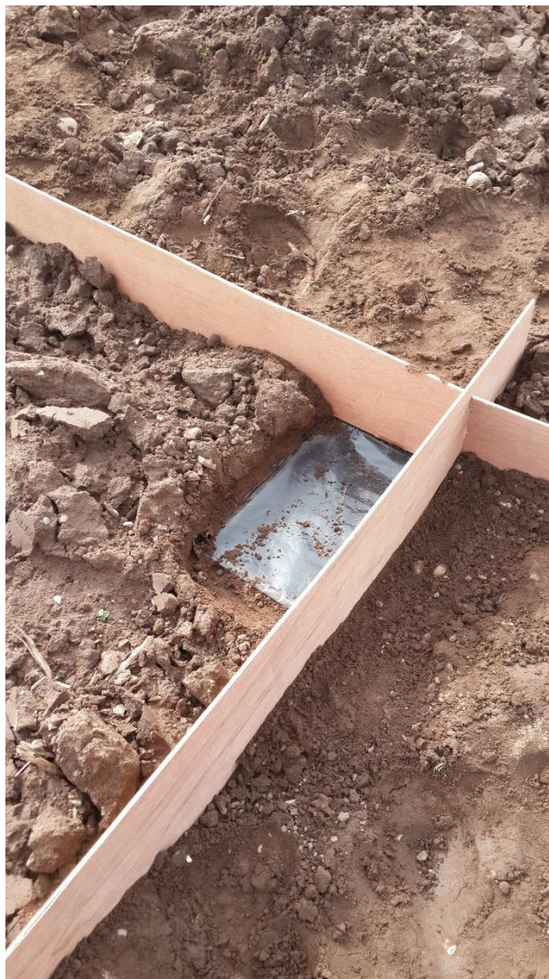
Figure 6. 12 Installation of the collector
