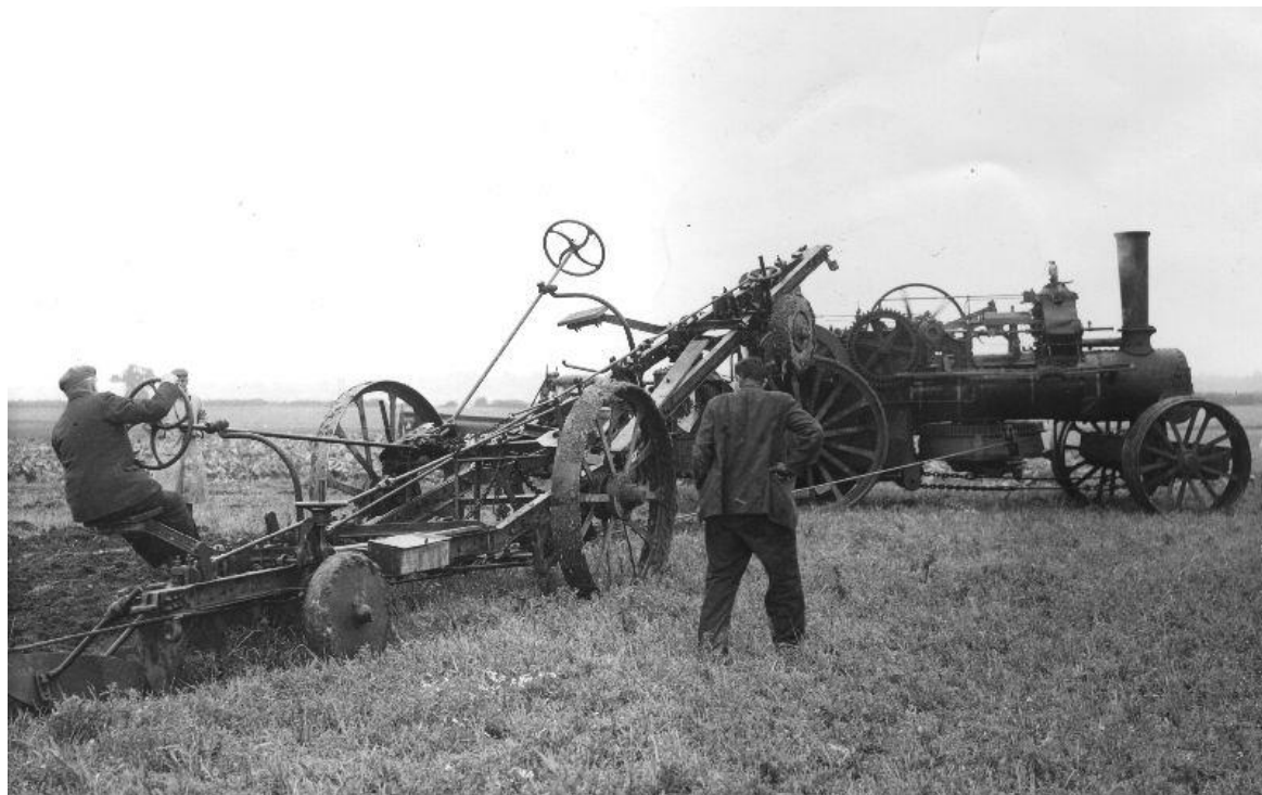
Figure 1: Early stationary tractor ploughing
