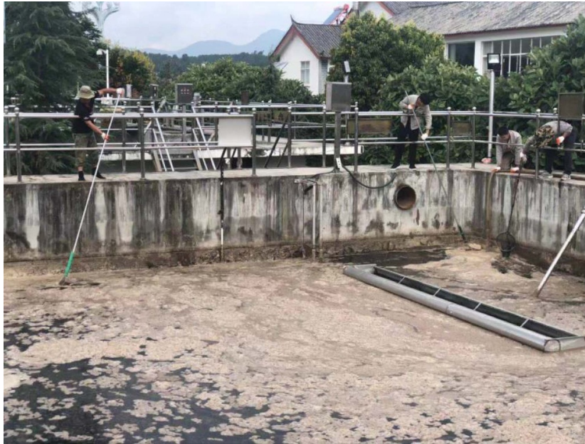
Figure 4. Floating oil and fat from kitchen wastes on the oxidation pond of a sewage treatment plant in Lijiang city, a tourism hot-spot in south China, following the implementation of the ASF control policy in 2019, which prohibited swill feeding to pigs. The table presents the mean total nitrogen (TN) concentration of the water in the adjacent river, which receives the effluents from the treatment plant, in 2017 and 2019.
