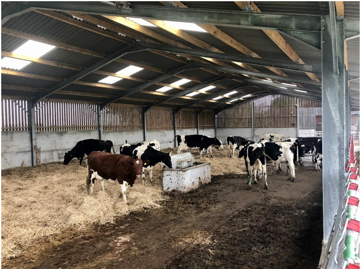
Figure 3.2.3: An example of a newly installed loose-housed 'fresh cow group' for cows 0-21 DIM, with locking head yokes at the feed barrier to allow for easy cow handling, and close to the milking parlour for minimal walking distance, e.g. on farm 1.
