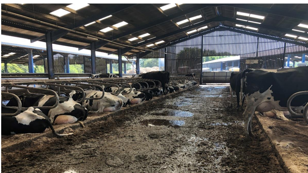
Figure 3.2.12: An example of a main milking group housed in a light and well-ventilated purpose-built shed designed with wide passageways (5.5m) e.g. on farm 18.
