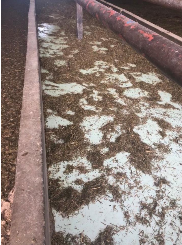
Figure 3.2.18: A feed trough with a resin floor for the main milking group, on e.g. farm 20.
