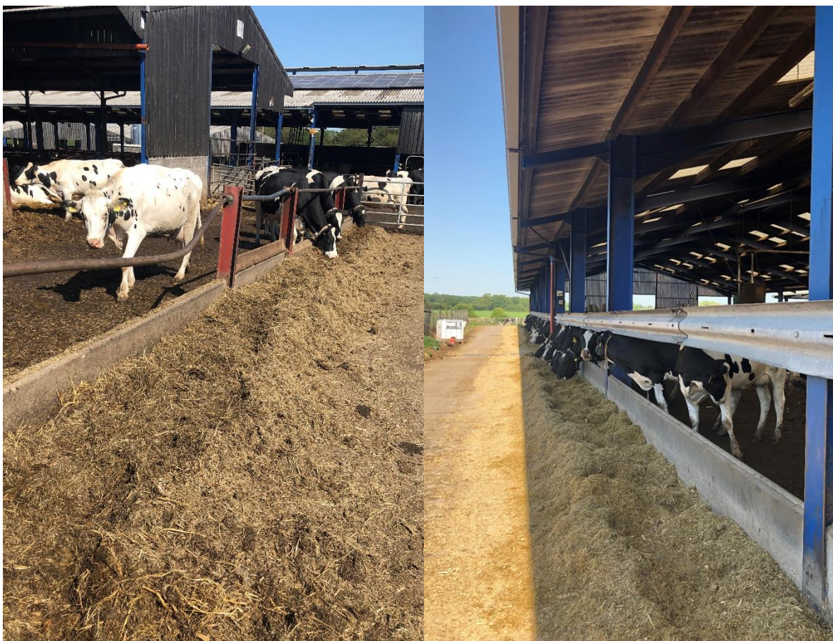
Figure 3.2.17: An example of a pre-calving cow feed barrier (left) where feed space and neck rail height did not meet recommendations, and a main milking group feed barrier (right), on the same farm (e.g. farm 18) where feed space and neck rail height met AHDB (2012) recommendations.
