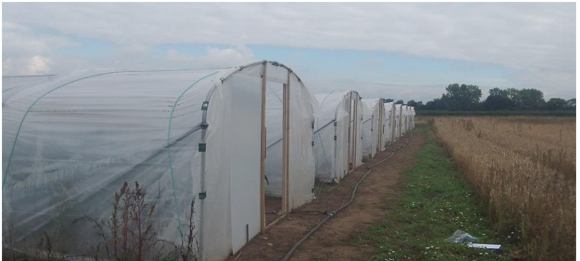
Figure 5.1.2. Front view of polytunnels showing doors and pipes for irrigation.
