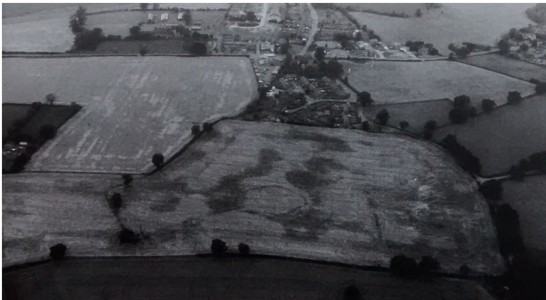
Figure 16. Aerial photography of the bridge site of the green cluster (source: English Heritage).
